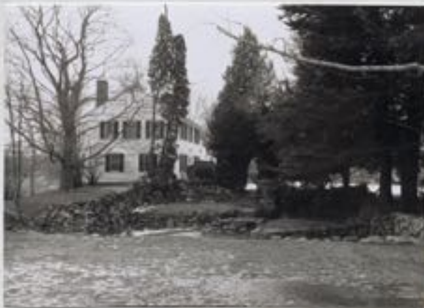
Photograph 63 View of Chaise House, looking north from sunken garden in 1989.
