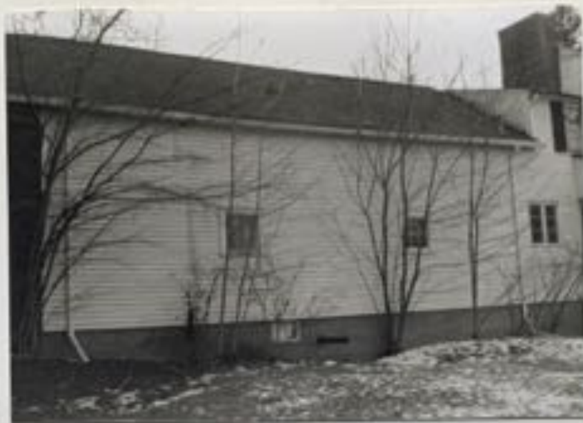
Photograph 33 Rear (west) elevation of the Corn Barn, 1989.
