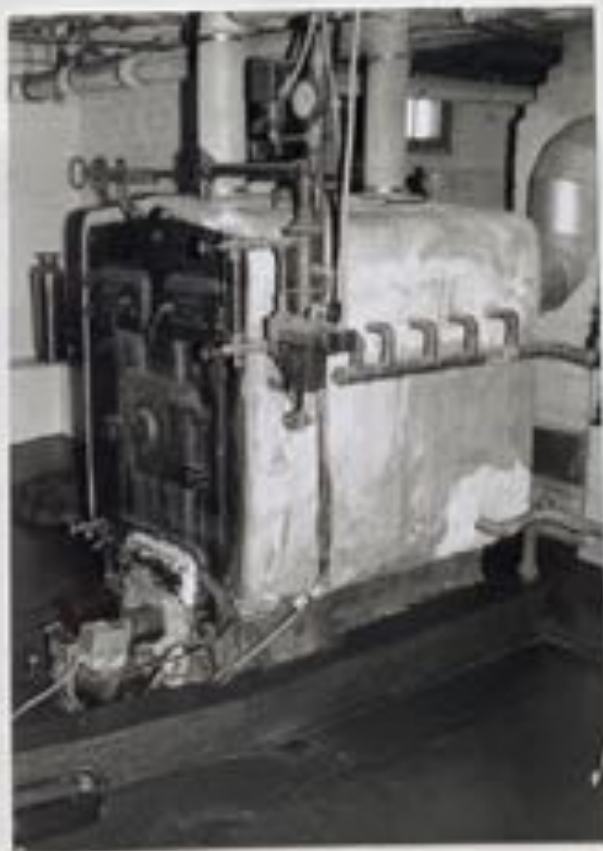
Photograph 68 Chaise house furnace, 1930, United States Radiator Corporation.
