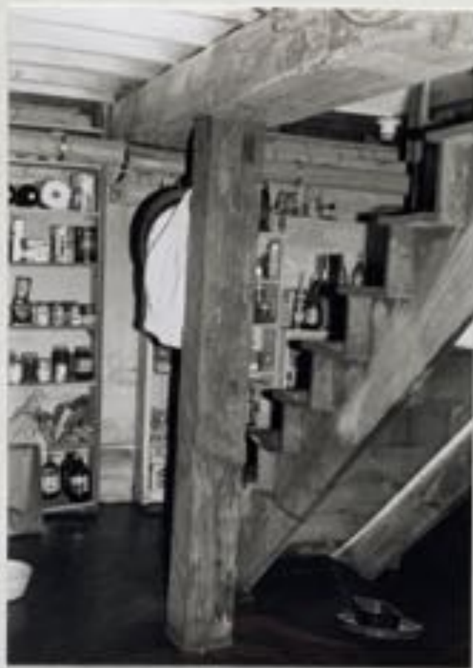
Photographs 9, 10, 11, 12, and 13 Timbers from original chaise house, reused as support posts, summer beams and sills in 1930 Chaise House basement.
