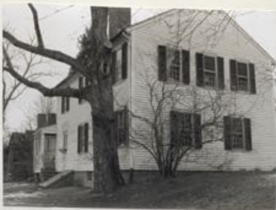
Photograph 39 Chaise House, south and west elevations, 1989.
