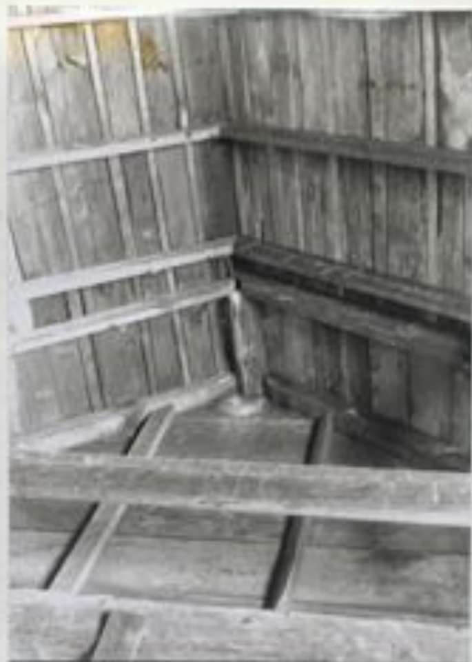
Photographs 20 and 21 North end of Corn Barn roof, showing original ridge pole extending through from the wood shed.
