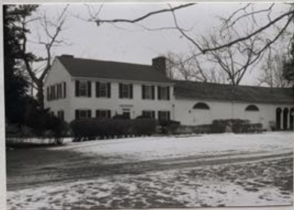
Photograph 4 Chaise House and Corn Barn, 1989.
