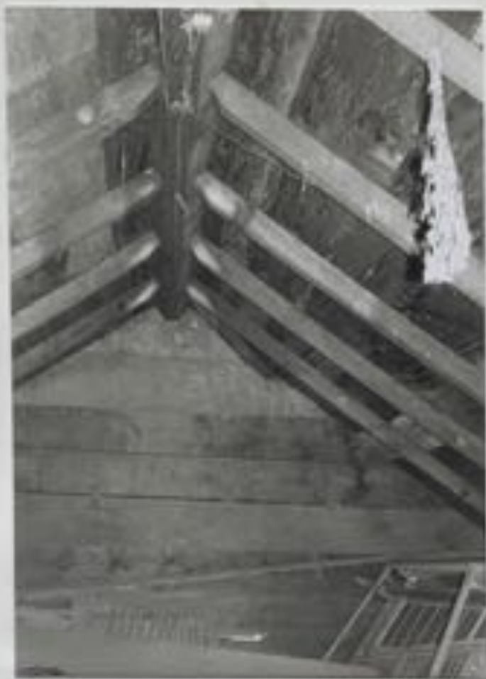
Photograph 26 South end of wood shed attic, showing original 1797 roof framing.
