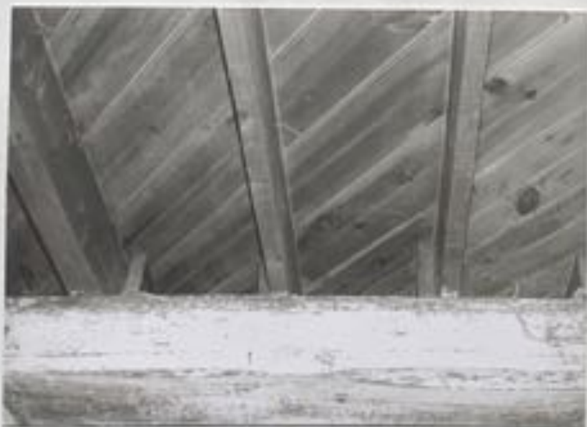
Photograph 61 New floor joists and subflooring under Chaine House.
