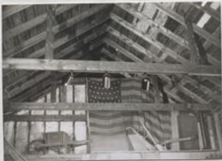
Photograph 34 Corn Barn roof framing, view facing south.
