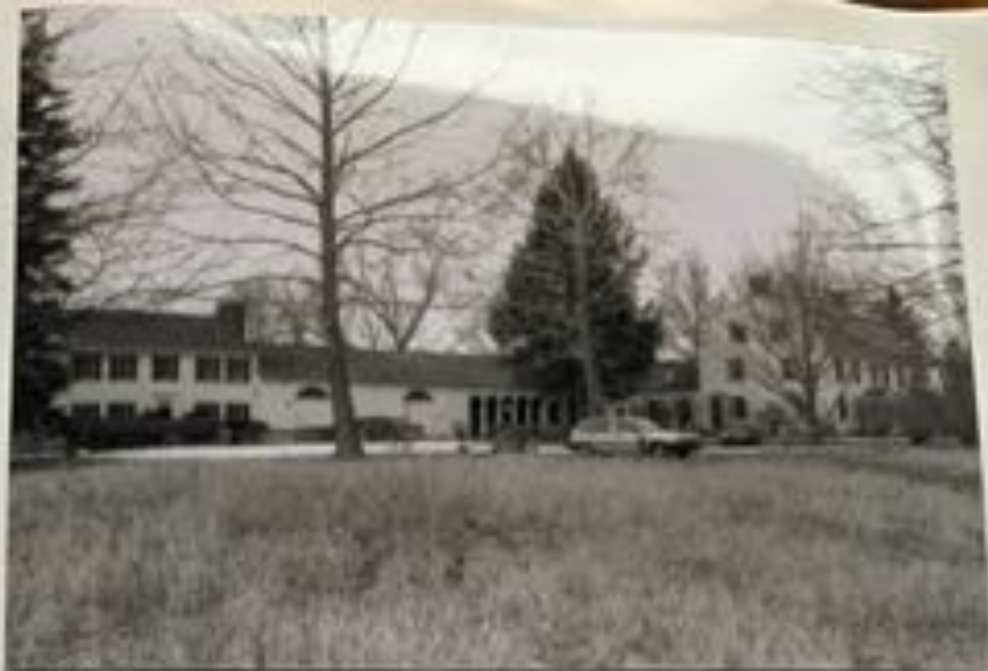
Photograph 1 Porter-Phelps-Huntington House, view looking north west, 1989. Chaise House at far left.
