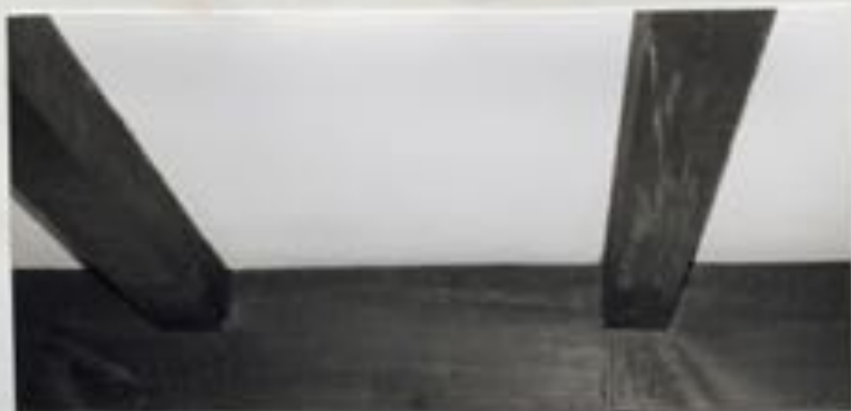
Photographs 56 and 57 Exposed framing in living room.
