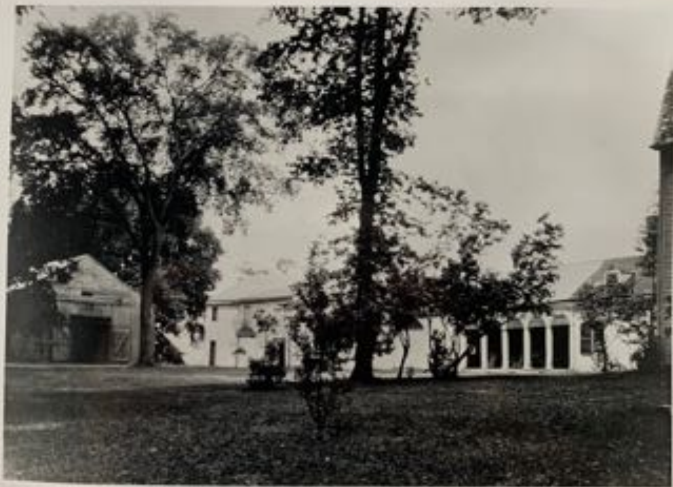
Photograph 2 Porter-Phelps-Huntington House, view looking south west, showing barn, chaise house, and sheds, taken August 1929. From James Lincoln Huntington Journal, page 109. Porter-Phelps-Huntington Family Papers, Box 80a.
