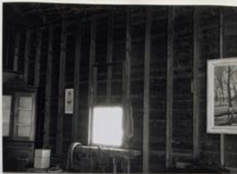
Photograph 36 West wall of Corn Barn, showing balloon frame construction.
