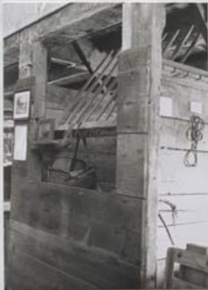
Photograph 15 Front end of chaise house stall, showing hay rack.
