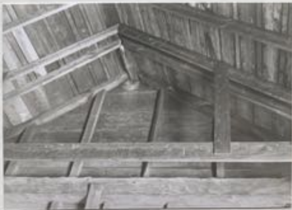
Photographs 20 and 21 North end of Corn Barn roof, showing original ridge pole extending through from the wood shed.
