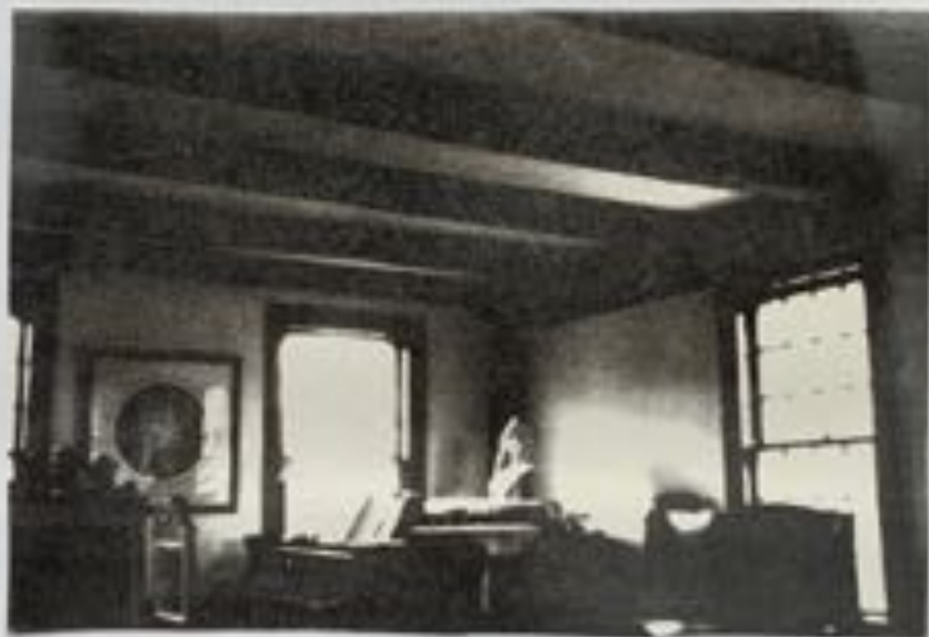
Photograph 55 South east corner of living room, showing exposed framing reused from original chaise house.
