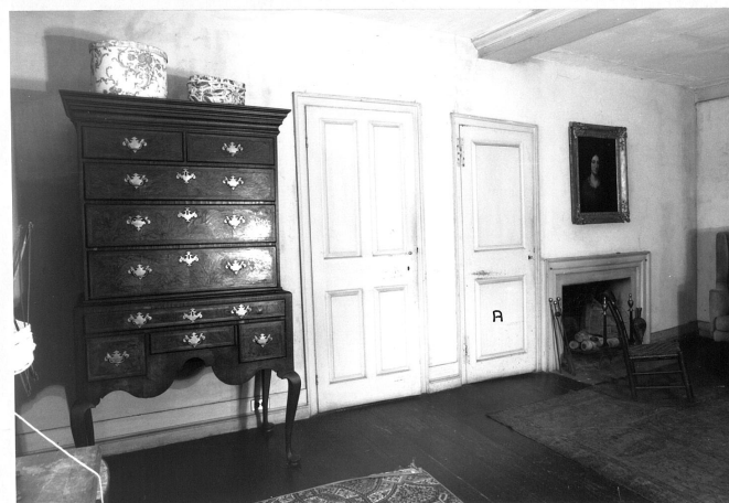
52. Southeast Bedroom, second floor, south wall; wall dates from c.1799, but door (A) was reused from an earlier location.
