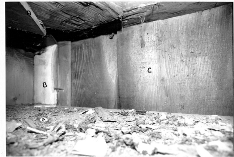
24. Attic floor cavity in location of original south chimney, showing summer (A), and casing cut to accommodate corner fireplace in southeast bedroom below (B).
