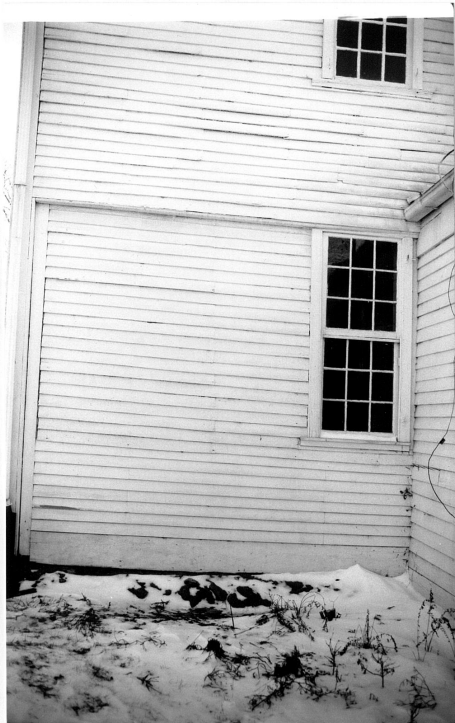
5. Main Portion, first story, west elevation, showing overhang.
