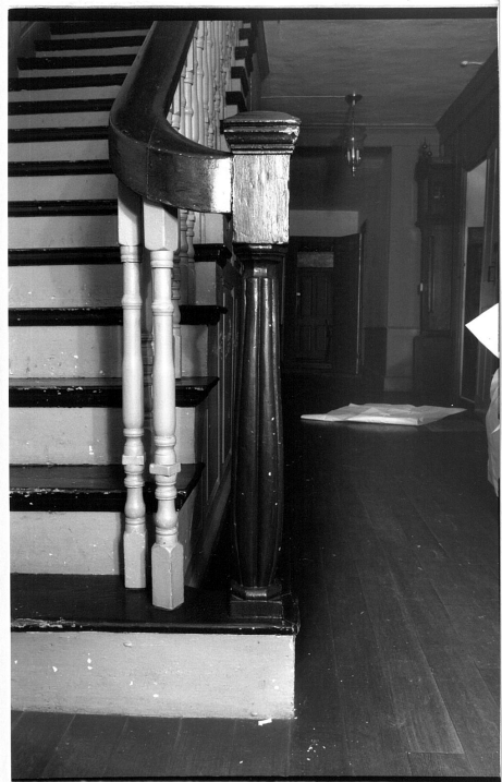
27. Newel and balusters, Main Staircase, central hall.
