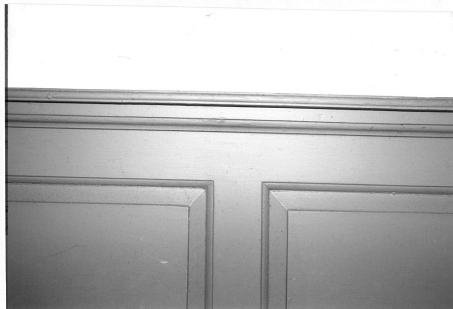
42. Wainscot and chair rail in Back Hall, east wall (above), west wall (below). The woodwork on the east wall was probably pieced together c.1799, while that on the west wall may date from the 1770's/80's.
