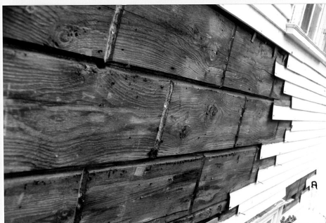
11. Rusticated Siding beneath clapboards on south elevation of Main Portion above door (typical); white paint visible in joints; overhang occurs at (A).
