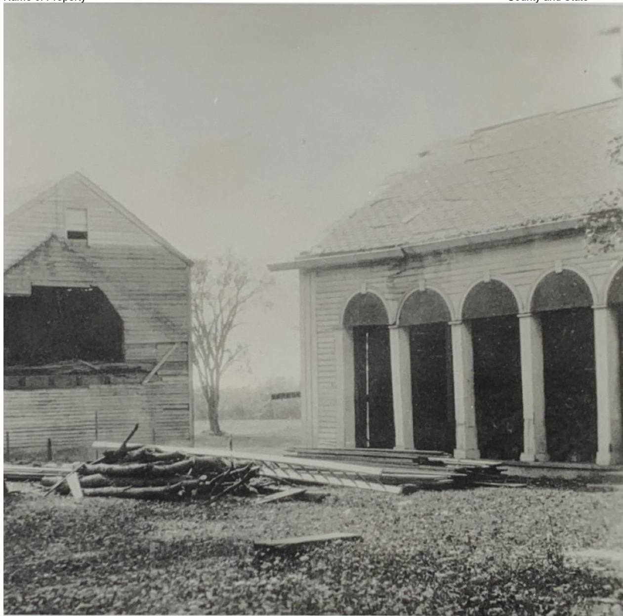
Figure 21: Reconstruction of the Corn Barn at Forty Acres Main House (HAD.319) in October 1928 showing the original 1795 carriage house (left) and Woodshed (right). Source: James Lincoln Huntington Journal, page 84.
